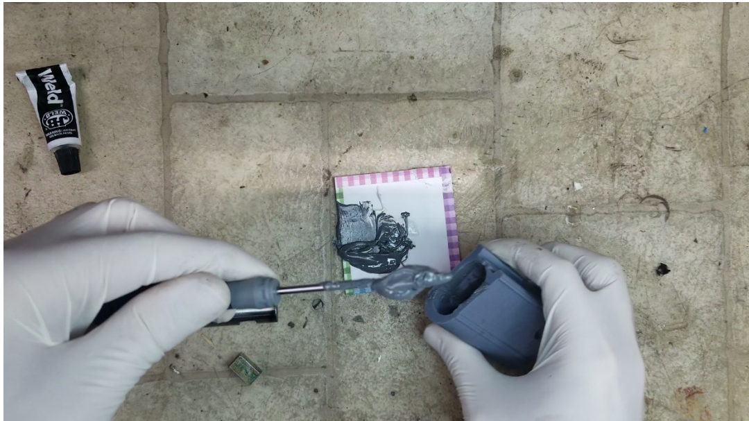
Apply JBWeld to the inside of the housing. Use your tool to spread it out.
