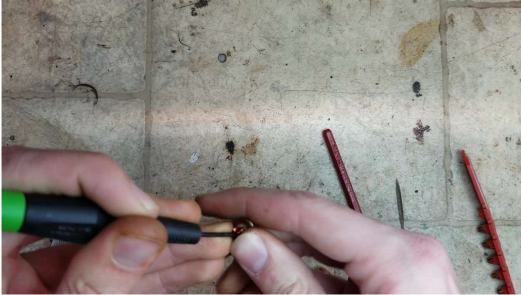
Step 5: Spreading the crimp. DO NOT insert your tool deep into the hole unless there is no gunpowder left.
